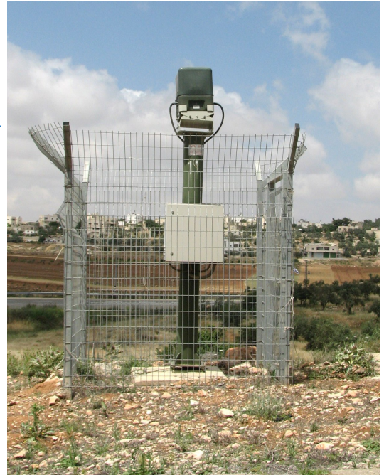
Motorola's MotoEagle Surveillance System radar station outside the settlement of Otnel.
